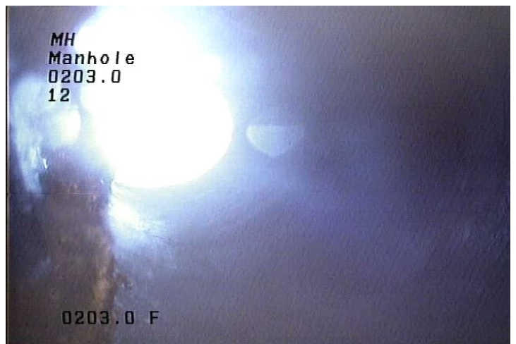
MH - Manhole @ 203.0 ft.
