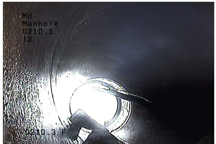
MH - Manhole @ 210.1 ft.
