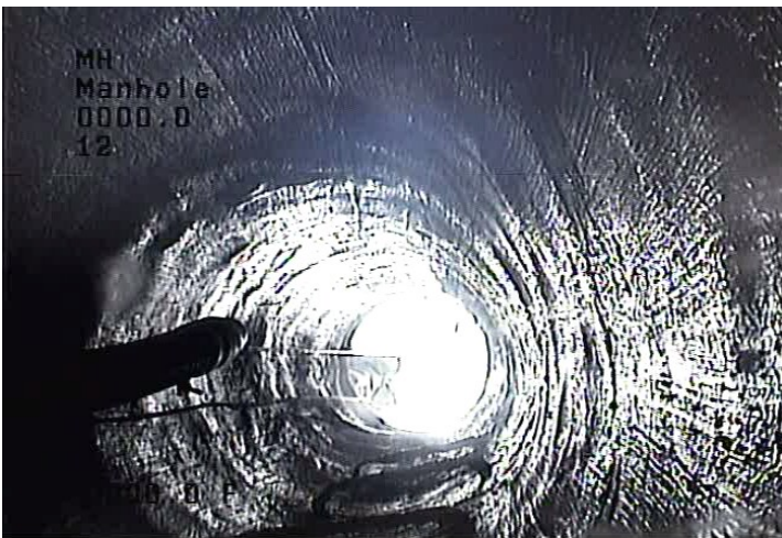
MH - Manhole @ 0.0 ft.
