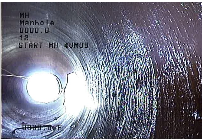
MH - Manhole @ 0.0 ft. START MH 4UM09
