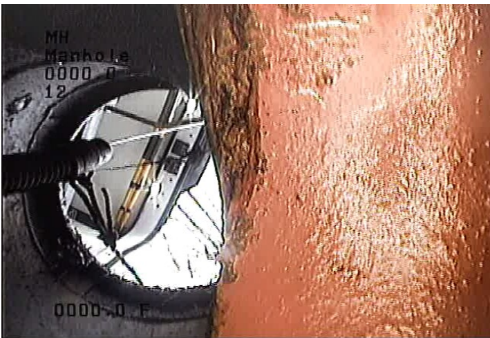
MH - Manhole @ 0.0 ft.
