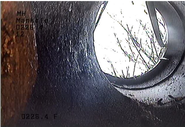
MH - Manhole @ 226.4 ft.
