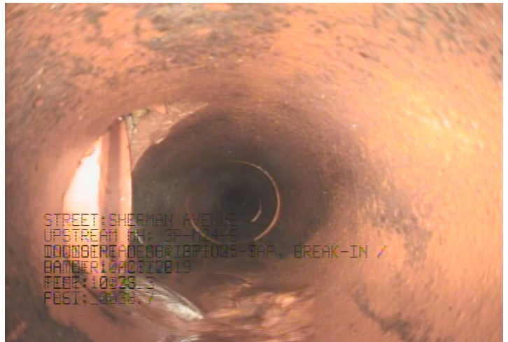
TBA - Tap, Break-in / Hammer: Active @ 38.3 ft.
