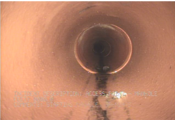
AMH - Access Point - Manhole @ 0.0 ft. Starting Manhole: 3P-M24-S
