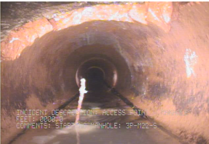
AMH - Access Point - Manhole @ 0.0 ft. Starting Manhole: 3P-M22-S
