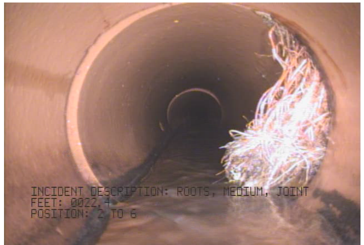
RMJ - Roots, Medium, Joint @ 22.4 ft.
