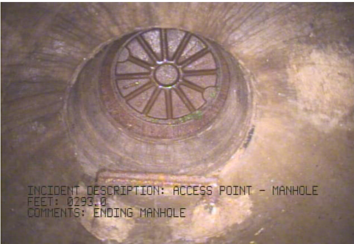
AMH - Access Point - Manhole @ 293.0 ft. Ending Manhole 3P-M22-S
