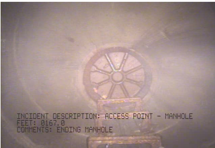
AMH - Access Point - Manhole @ 167.0 ft. Ending Manhole
