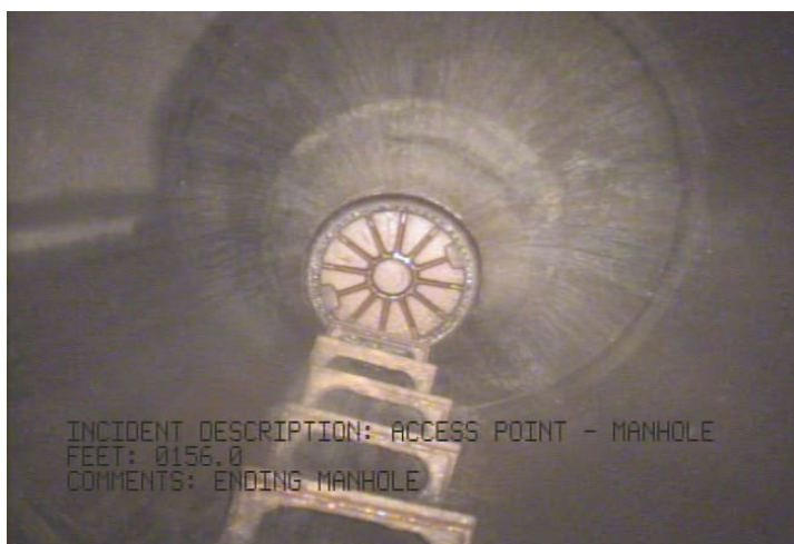
AMH - Access Point - Manhole @ 156.0 ft. Ending Manhole 3P-M20-S
