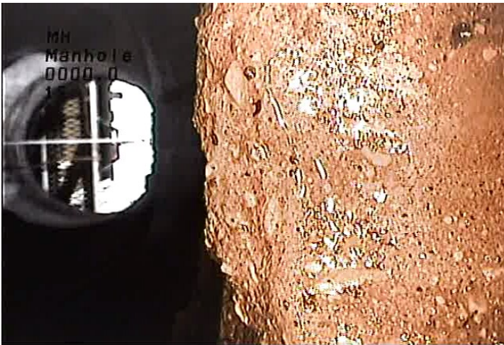
MH - Manhole @ 0.0 ft.
