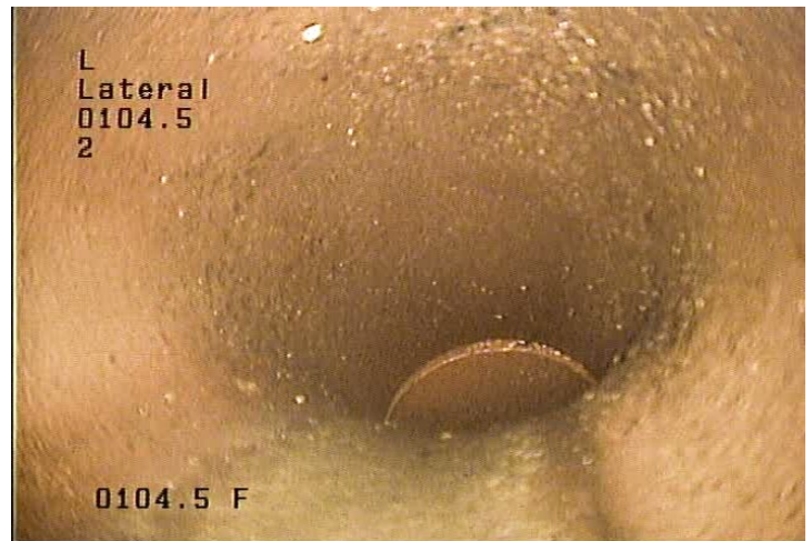
L - Lateral @ 108.5 ft. STUB
