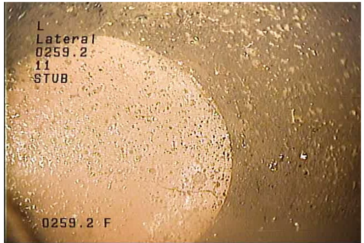
L - Lateral @ 259.2 ft. STUB
