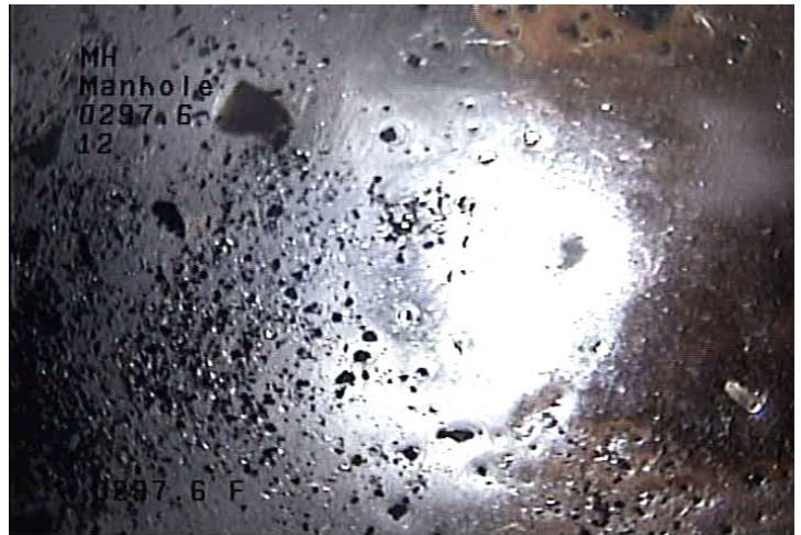
MH - Manhole @ 297.6 ft.
