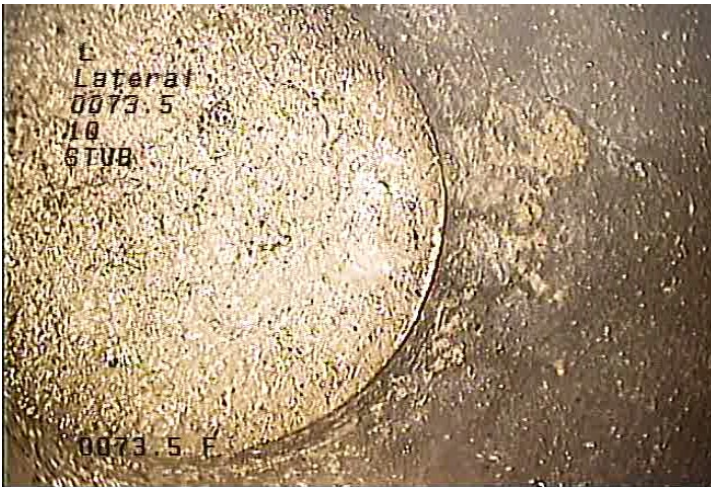
L - Lateral @ 73.5 ft. STUB
